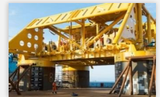
Åsgard Subsea Compression
